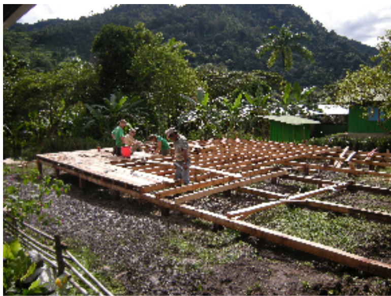
The work we have completed in Phrase I before we left
